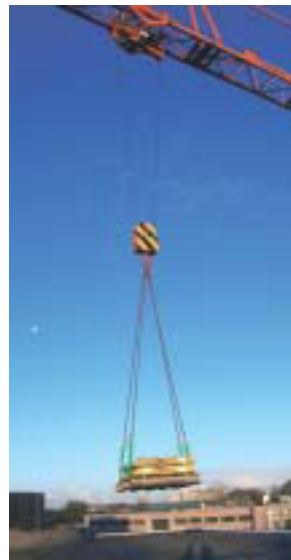
Lifting BIBO® Blocks/Corners into position by crane.
