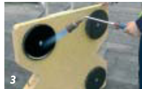
Preparation of a BIBO® Block and a plain bitumen roof surface.
