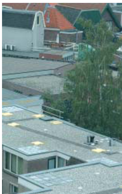
A typical, completed BIBO® Lifeline installation. Once the work is finished, the lifeline is detached from the BIBO® Blocks/Corners and stored away with safety harnesses, lanyards, etc.
