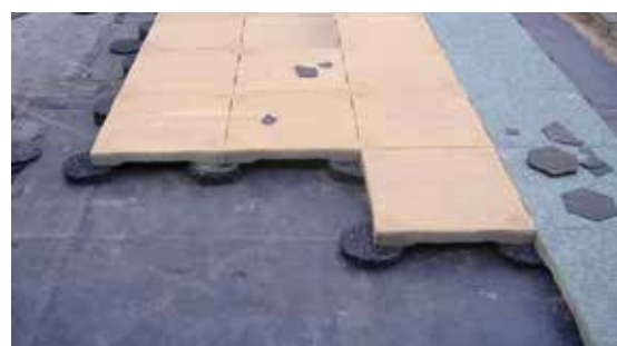
Dreen® Slab: Laying fixed height system
