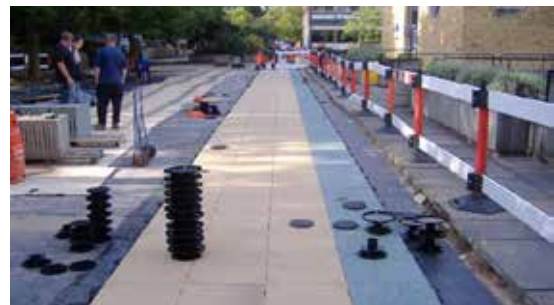
Dreen® Slab: Laying adjustable height system
