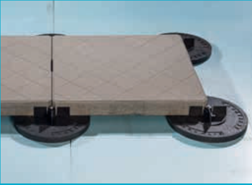
The slabs are laid on the pressure distributor pads
